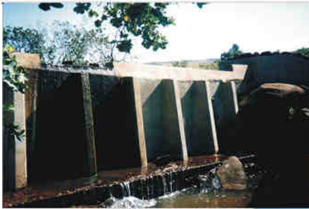
Weir for rural domestic water supply near Paulpietersburg.
