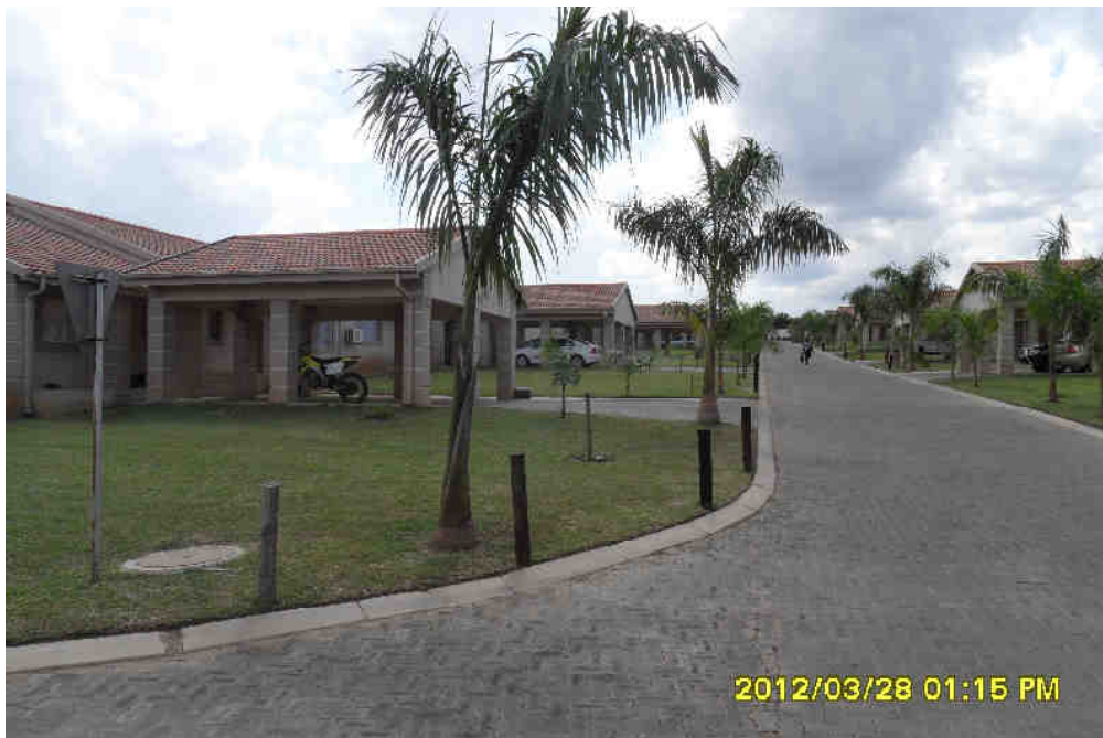
PALM VILLA PONGOLA : 100 SEMI ECONOMICAL HOUSING UNITS
