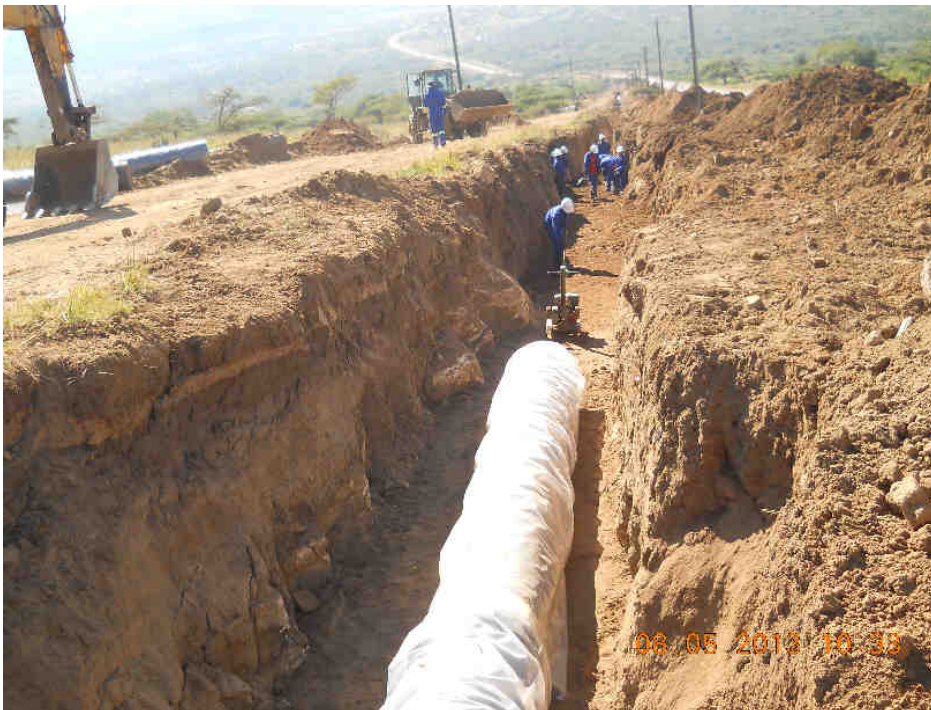
USUTHU WATER SUPPLY 600mm DUCTILE IRON PIPELINE
