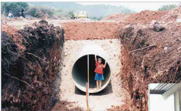
Bulk water supply scheme at Mkuze. 1,4m diameter 7km GRP pipe including 640kw pump station and 50 000 m 3 balancing dam.
