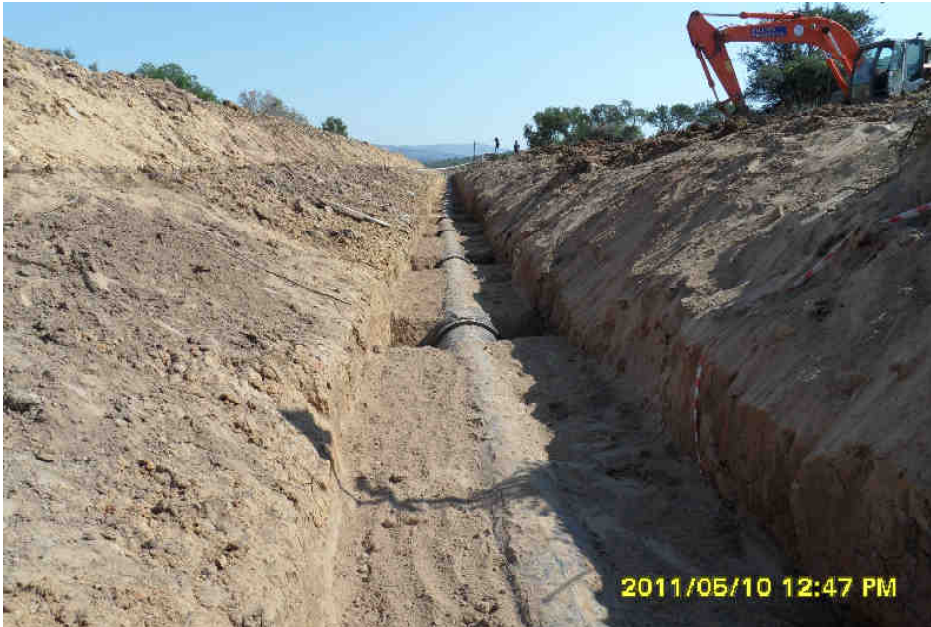
USUTHU WATER SUPPLY 700mm DUCTILE IRON PIPELINE
