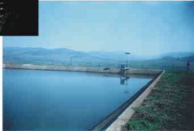
Bulk water supply scheme at Mkuze. 1,4m diameter 7km GRP pipe including 640kw pump station and 50 000 m 3 balancing dam.
