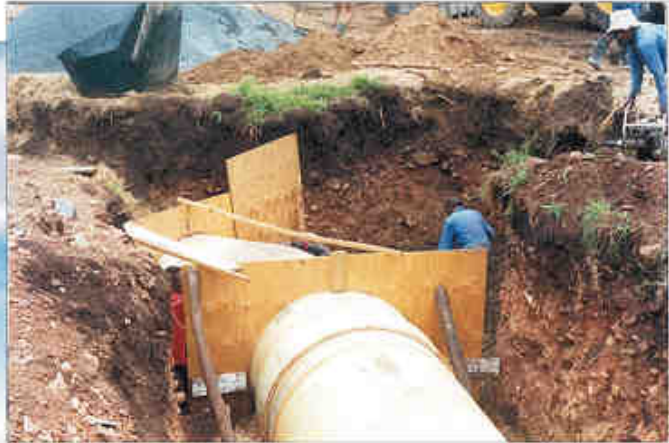
Thrust block shuttering for 7km 1,4m diameter GRP pipe at Mkuze.
